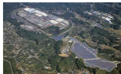
Suzuki Makinohara Solar Power Plant
