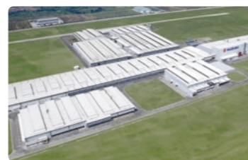
30 PT. SUZUKI INDOMOBIL MOTOR (Cikarang Plant)
