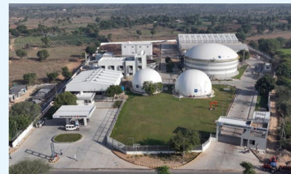
BANAS SUZUKI BIOGAS PLANT
